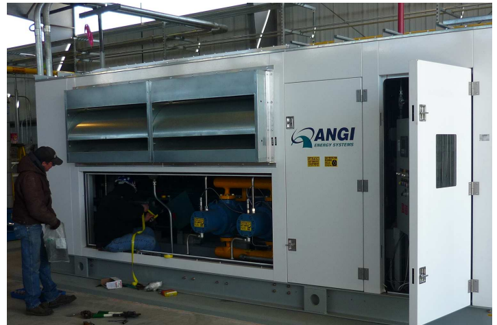
As Michigan’s largest producer of alternative fuel , Blue Water Area Transit uses a wide range of equipment that includes this natural gas compressor. The agency has produced compressed natural gas to fuel its buses since 1996.
